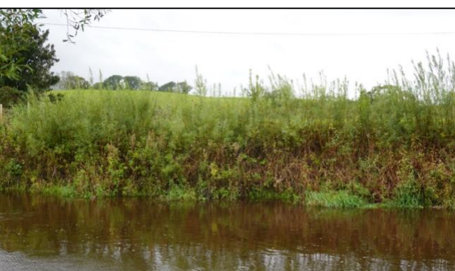
Figure 4: the stabilised banking in autumn 2025
