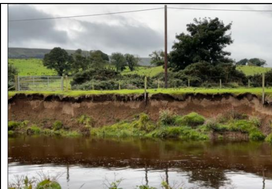
Figure 1: The banking prior to any works
