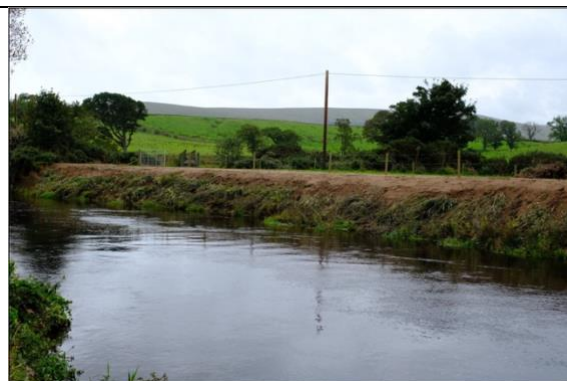
Figure 2: The banking immediately after work in September 2023
